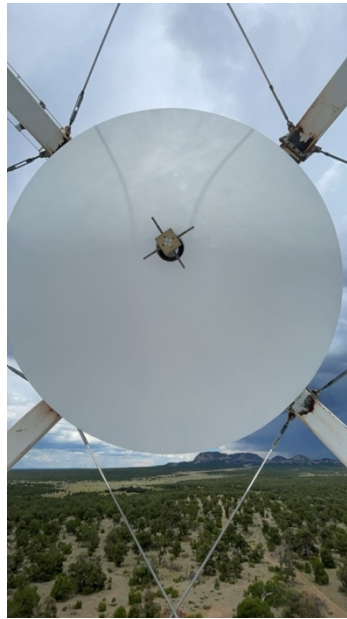
Los Alamos Subreflector painting in situ (left: before, right: after). Measurable gain improvements were seen following this major maintenance visit.
