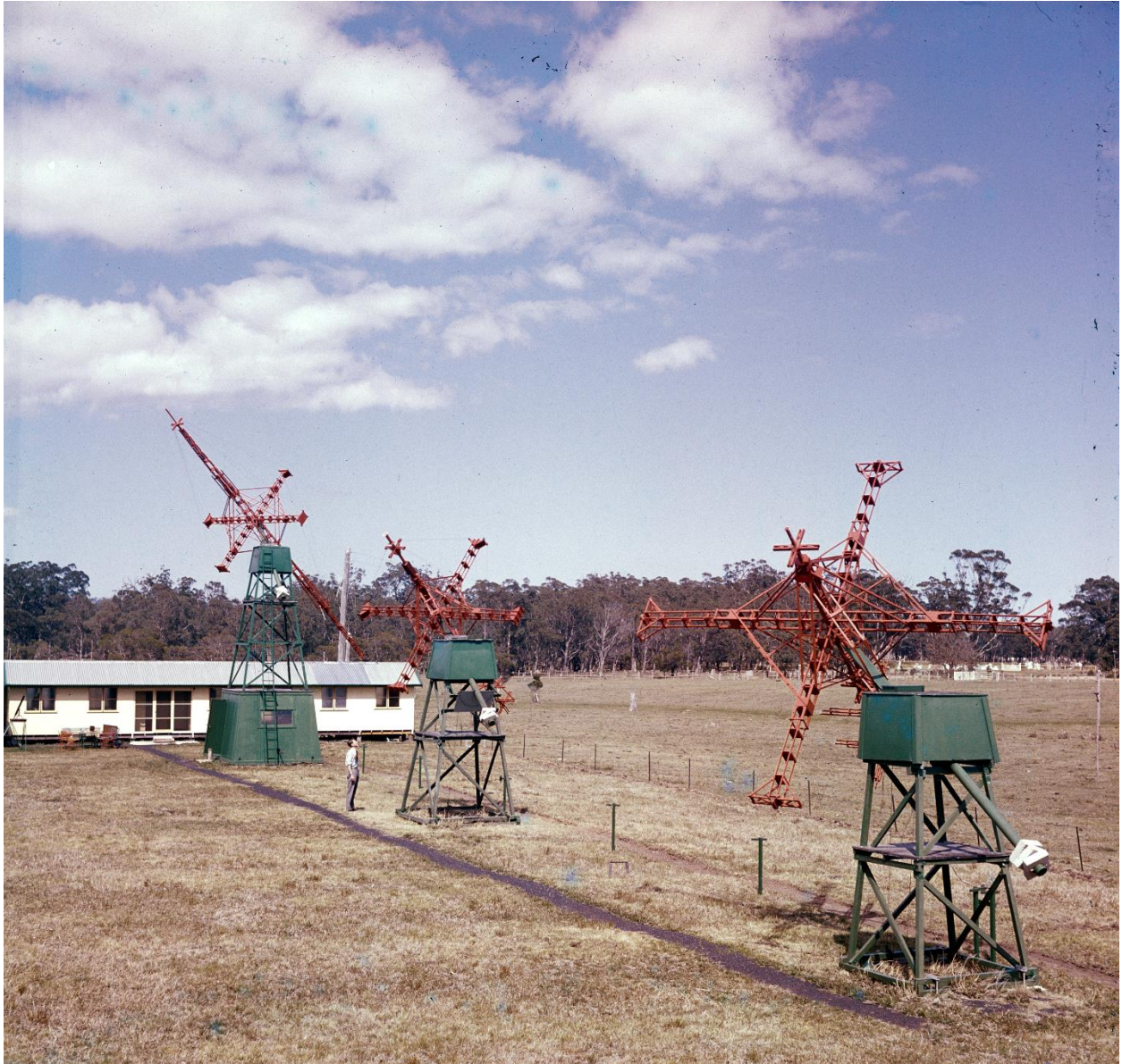
Fig. 25 The epoch of the photo is likely from the era 1958 to 1960- the initial three elements of the dynamic spectra instrument – from left 40 to 75 MHz, 75 to 140 MHz and 140 to 240 MHz. Credit: CSIRO Radio Astronomy Image Archive R12429-1 (1980).
