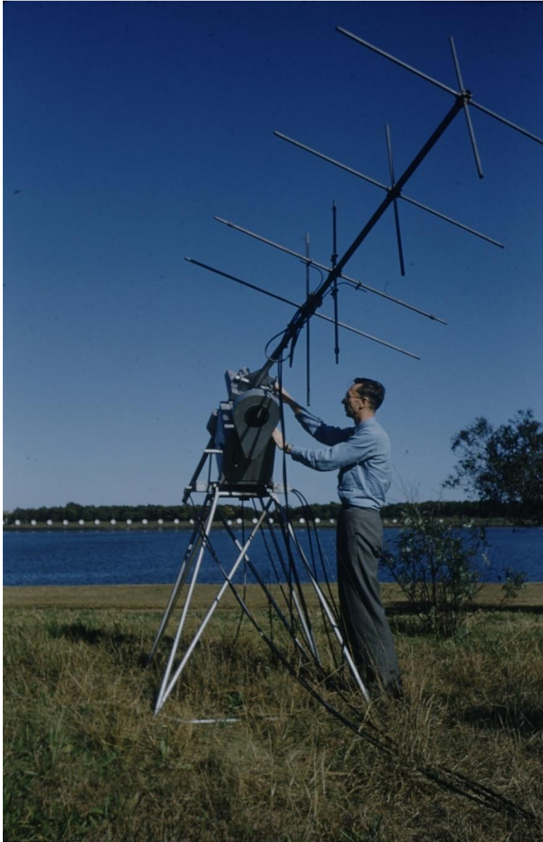
Fig 22 Fritz Goro image from March 1951 of Pawsey with the total power 98 MHz aerial at Potts Hill. The EW arm of the grating array is seen in the distance on the south end of the reservoir at Potts Hill. See Additional Note No 1 in NRAO ONLINE 23 ("Fritz Goro, Life Magazine Photographer at Potts Hill, Dover Heights, Mt. Stromlo and Harvard University, 1951. Photographs of RPL, ANU and Harvard Scientists.") Credit: Getty Images, Fritz Goro, The Life Picture Collection, licensed by Getty November 2021 / Licence organised by Shutterstock, Inc., New York, NY (5 Nov 2021) Original , Premium Editorial All Media
