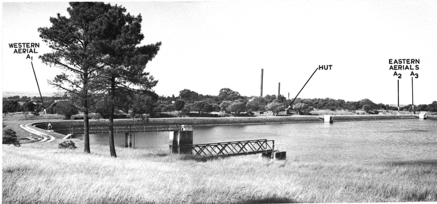
POTT'S HILL INTERFEROMETER SITE LOOKING NORTH-EAST PLATE I
