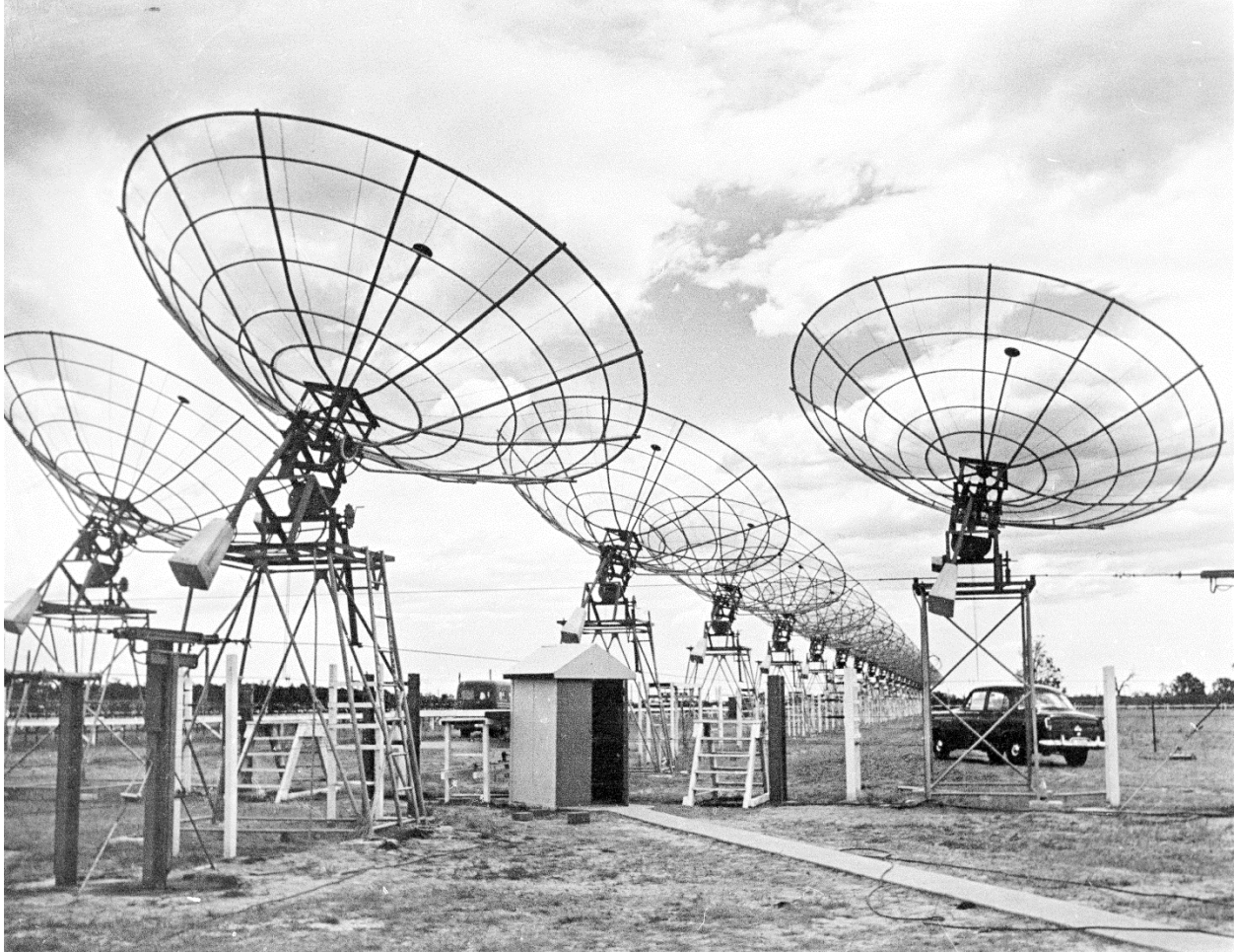
Fig. 20 Centre of the Fleurs 1423 MHz array, the central 5.8m aerials are shown , in the distance the west arm. Credit: CSIRO Radio Astronomy Image Archive B5372-7
