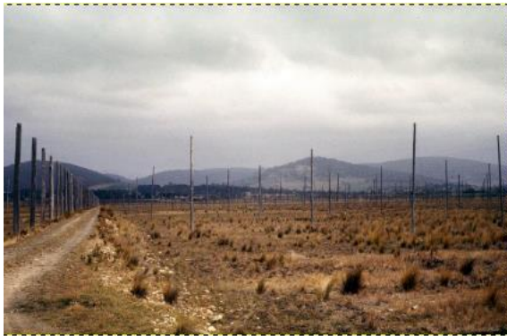
Left: poles of the Llanherne Low Frequency Array near Hobart, Tasmania. Operating at frequencies between 2 MHz and 35 MHz, this was one of the University of Tasmania's major low-frequency instruments. It was used from 1972 to the early 1980s to record bursts of decametric bursts from Jupiter and map the radio sky at low frequencies [46]. Credit: the estate of Grote Reber. Right: the University of Tasmania's 26-m antenna at Mount Pleasant Observatory. Credit: Jim Lovell
