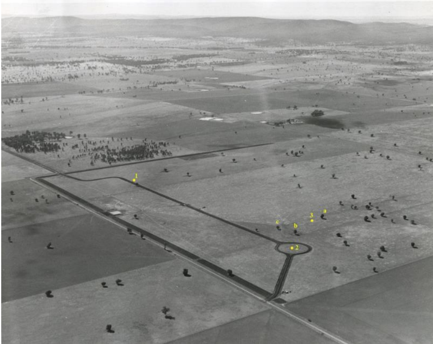
Fig. 15 PEG EVENTS 1, 2 and 3. An aerial photograph showing the positions of all three peg events (1,2 and 3) and the “famous” a,b and c trees. The time of this photo is uncertain, likely in the time frame October or later in 1959 to early 1960. Excavation for the tower began in late September 1959. The MAN crew from Germany arrived in September 1960.
