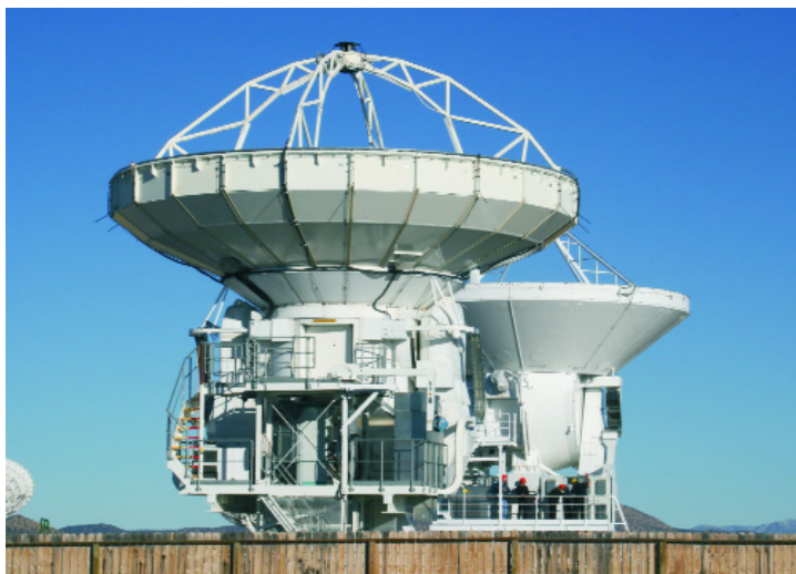
Figure 2. The prototype ALMA antennas (VertexRSI, foreground; AEC, background) stand ready for prototype system integration near the Very Large Array in New Mexico.
