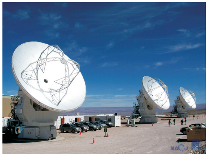
Figure 2. Three Melco antennas under operation at the OSF. On the right is Melco unit-1, the most thoroughly tested of these antennas. Photo courtesy NAOJ.
