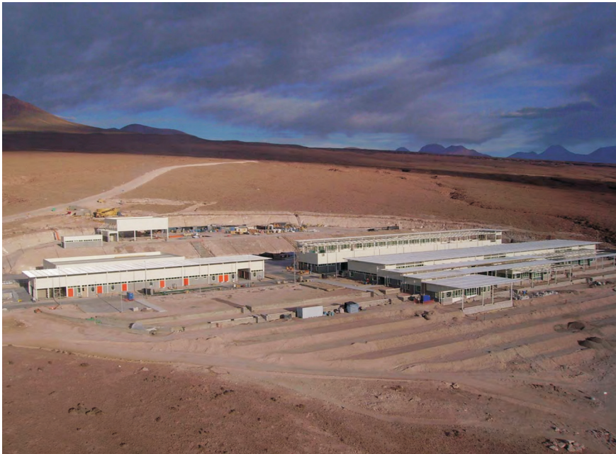
Figure 4. The Operations Support Facility Technical Building complex, seen from the holography tower in mid-October, is nearing completion. The warehouse is on the left, with offices and labs on the right. The transporter shelter can be seen in the background.
