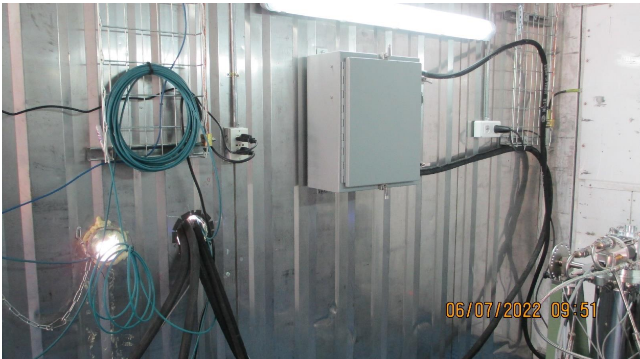
Picture 32: Charcoal Trap Enclosure Mounted on the Container Wall, the Helium Lines Come from the Compressors on the Roof
