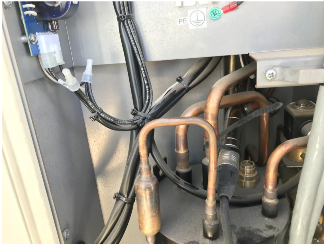
Picture 41: Installation of the condenser Microphone Inside the Sumitomo Outdoor Enclosure
