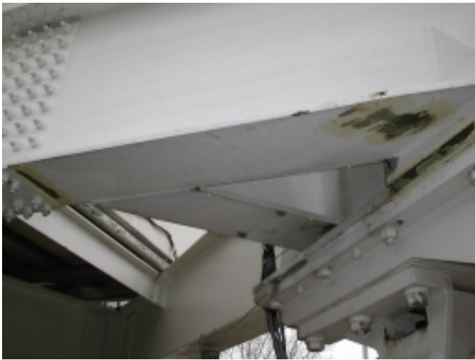
Figure 6: Pedestal Structure
