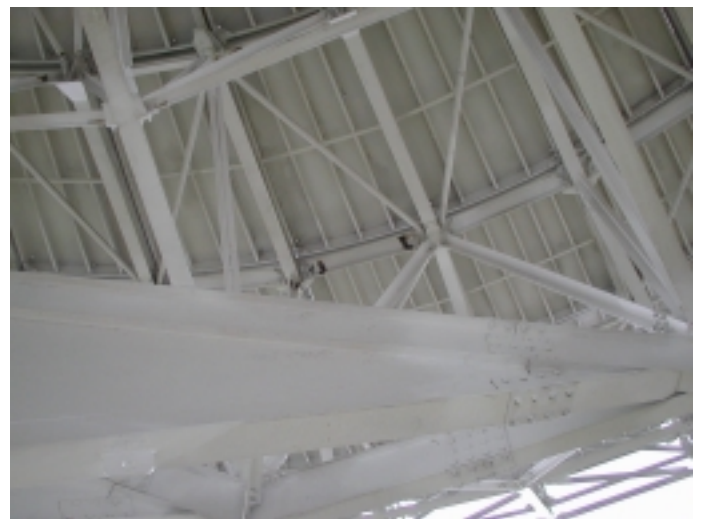
Figure 10: Backup Structure
