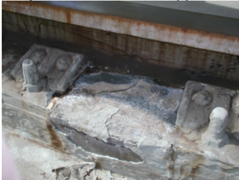
Figure 4: Grout Failure
