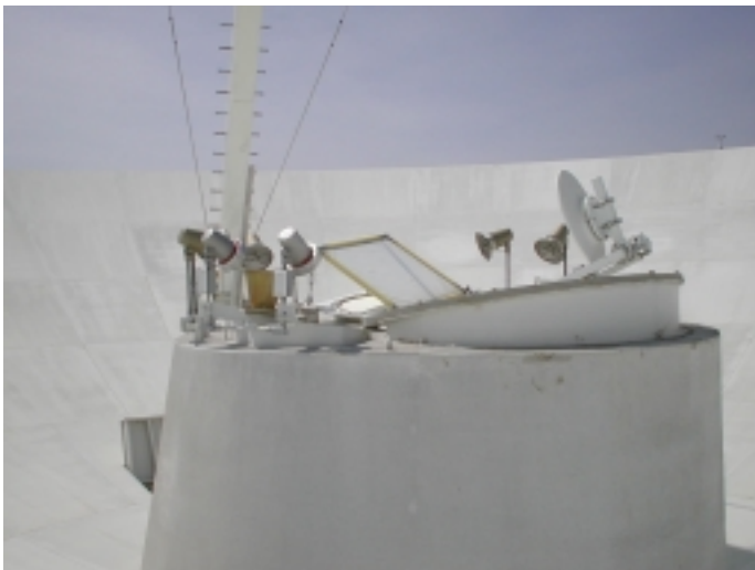
Figure 13: Feed Cone
