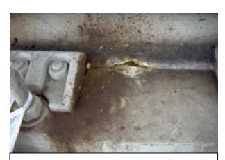
Figure 4: Grout failing under Vulkem
