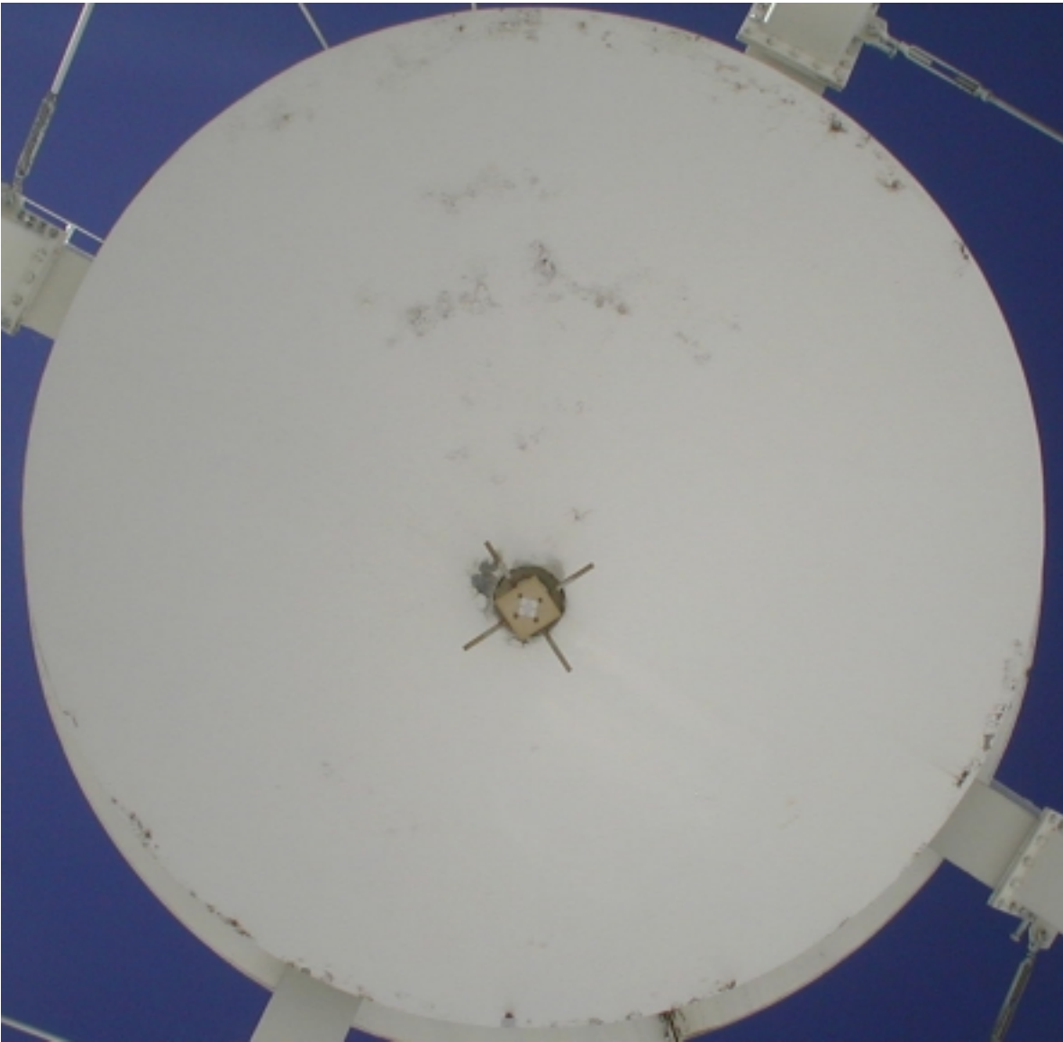
Some of the paint on the subreflector is peeling.
