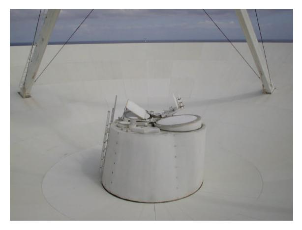
Feed cone insulation, ellipsoid reflector and dish panels are in good condition. Quad legs and guy wires have a little surface rust.
