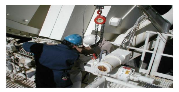
Elevation motor # 1 was replaced. The elevation bull gear is well lubricated.
