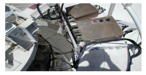
FRM motors to j-box cable connectors were replaced. As were the j-box to j-box connectors. The focus flex shaft and a bellows were also replaced.
