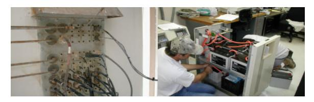
The ellipsoid reflector signal/power cable connectors on the vertex room baulk head were replaced. The station 12.5kva UPS batteries were replaced.
