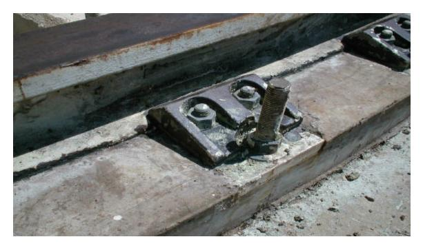
A typical rail clip with vulkem scraped off. Grout is in good condition. Site techs will follow up with chem prime paint on clips and splices as needed.
