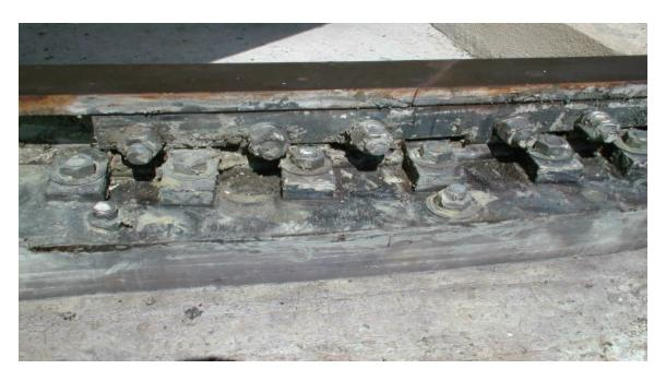
Rail splice with vulkem scraped off. The maintenance team and site techs were able to remove most of the vulkem from the rail during the visit. The rail, clips, and splices are in good condition.
