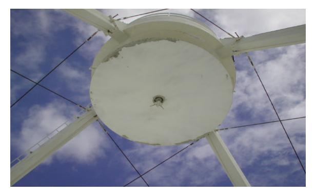
Subreflector has some peeling paint on the outside perimeter,  $\sim 3$ " strip.
