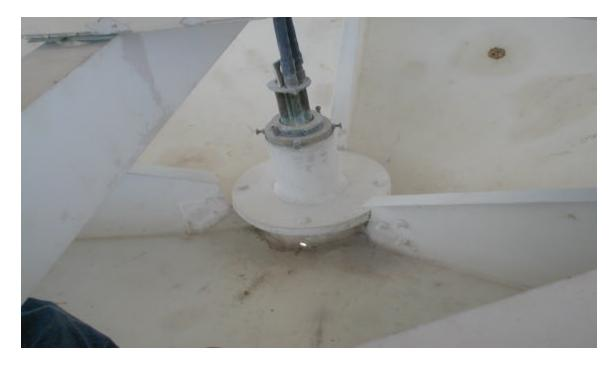
Subreflector drain holes are clear. The di-pole is in good condition but slightly corroded. 90/50cm FE cables are in good condition.
