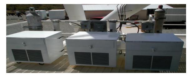
The cryo compressors are in good condition. Shown here with fresh paint.
