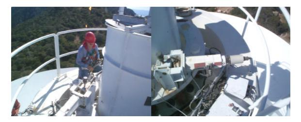
Duane greases the focus flex shaft. FRM is well lubricated and all j-boxes, cables, and connectors are in good condition. During the FRM PM a bellows was replaced. The focus flex shaft was replaced 2 months earlier by the site techs and not replaced by the maintenance team. The focus motor encoder coupling modification had been previously installed by the site techs.
