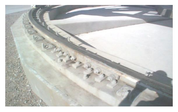
A typical rail splice. Rail splices and vulchem are in good condition.
