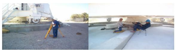
Ramon measures AZ #1&2 drive wheel alignment. The rail was measured.
