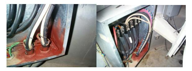
Inside the pintle bearing room power panel Bob found a ground terminal block severely corroded. The terminal block was cleaned and then sealed with primer. The antenna cable wrap and cables are in good condition.
