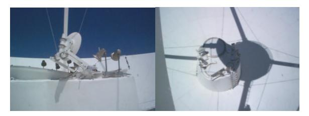
A spring was replaced in the ellipsoid actuator during alignment. Ellipsoid is in good condition. Feed cone FE windows and heaters are in good condition.
