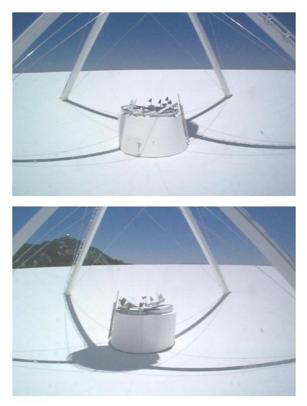
Feed cone insulation is in good condition. Dish panels, and the dish panel's paint are in good condition. Quad legs and guy wires are in good condition. Page 5
