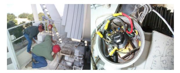
Elevation #1 and #2 motor gearbox rubber couplings (spiders) were replaced. The elevation gearbox heaters were wired in series. This was corrected to parallel and tested. The elevation bull gear is well lubricated and in good condition. Paint in the elevation platform area is in good condition.
