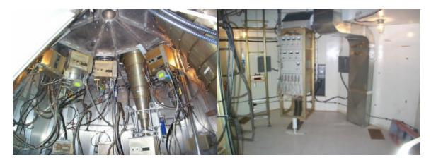
Feed cone & Vertex room. FE and rack cables are neat, orderly and secure. Page 4
