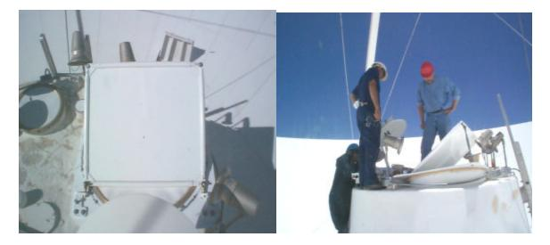
Dichroic reflector is in good condition except for a small delaminating blister in the center running verticality. The dichroic panel and ellipsoid reflectors were both realigned. Notice the feed cone is need of painting. Page 3
