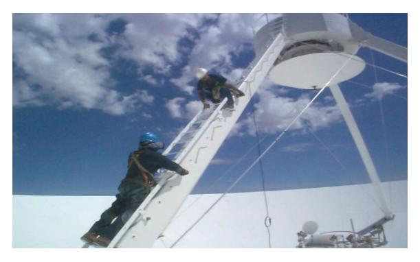
Ramon and Steve installing a new latter and fall arrest on the quad leg. The site techs were trained on using the new Sellstrom fall arrest.
