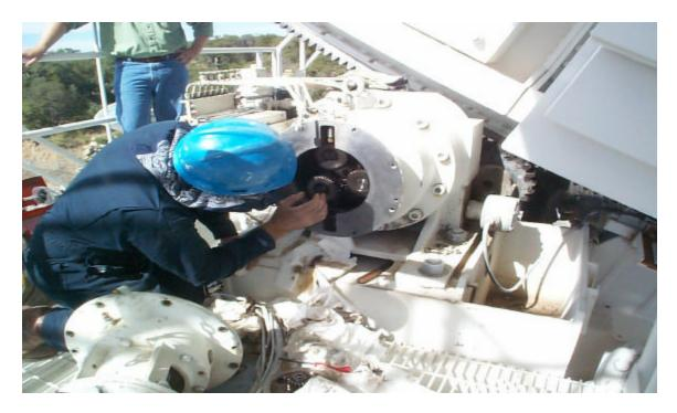
Elevation #2 gearbox pre-load inspection.
