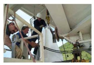
It was not possible to gain access to a large press on the island of St. Croix, so instead of risking the possibility of not being able to remove the old bearing from the bearing pillow block, a new elevation pillow block was fabricated and installed with the new bearing.
