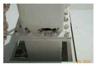
This picture shows a hole that has corroded all the way through the quad leg of the antenna. The steel on this side of the quad leg has completely failed due to this corrosion. The reason that the corrosion is so bad on this part of the quad leg is that water runs down the inside of the quad leg and pools on an internal lip in the quad leg. This quad leg should be repaired during the next maintenance visit.
