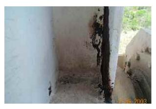
The major structural elements of the antenna were not severely corroded except for one of the beams that connect the dish to the elevation axle. Approximately 20% of the flange thickness has corroded away. This beam is in a pocket on the up side of the antenna where water collects. It will be very hard to drill a drain hole in this pocket. Therefore, the site techs should "Chem Prime" and paint these areas carefully.
