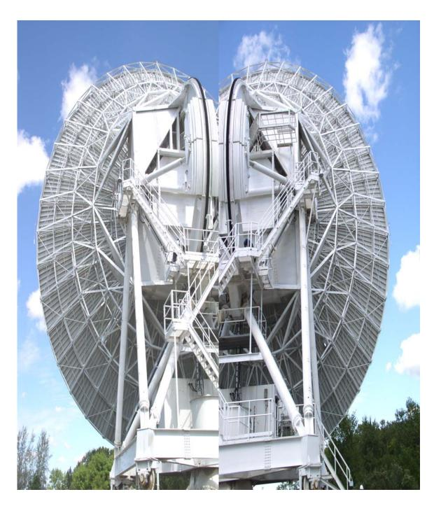
The antenna has alot rust and peeling paint almost everywhere you look. This summer the Site Techs should clean up and spot paint affected areas they can safely get to with chem prime. VLBA OPS should also dump water out of the antenna before an observation as recommended by Ramon and Jon for the SCVLB antenna.
