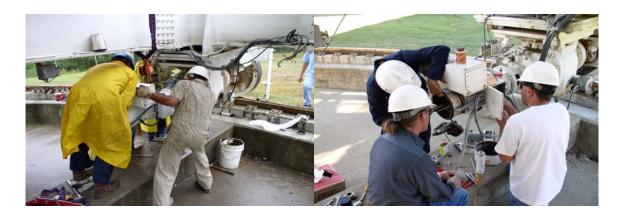
AZ #2 motor was replaced. AZ# 1 rear motor bearing seal was replaced.
