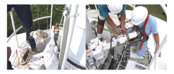
The FRM INA bearing zirks were installed. A 2<sup>nd</sup> screw and guide rod bellows were replaced during the FRM PM. Both focus motor encoder couplings were broken. These were replaced with the new encoder coupling modification. Apex j-boxes and cables are in good condition.
