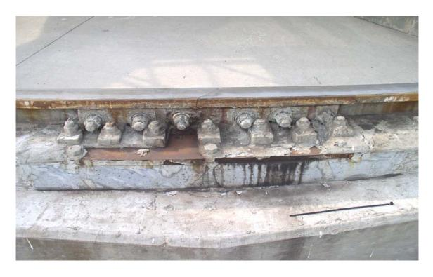
Vulchem is rapidly deteriorating from this rail splice and all the others.
