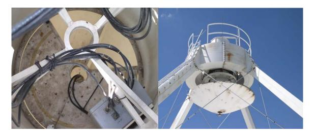
90/50 FE cables and connectors are in good condition. Subreflector drain holes are clear. Dipole is in good condition. Apex has lots of surface rust.
