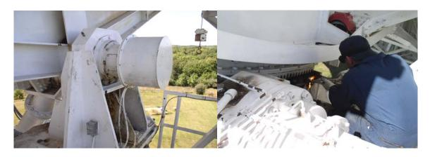
Elevation bearing grease trays were installed. A new stow pin tray and interlock switch were installed.
