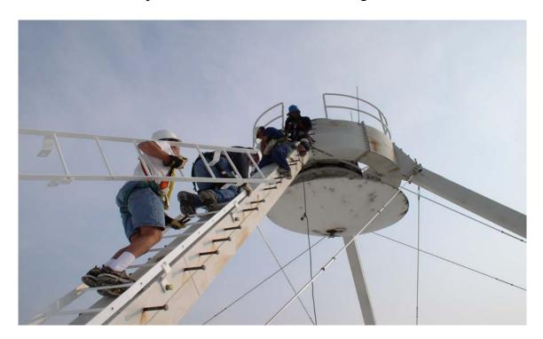
A new ladder and fall arrest was installed. Techs were trained on using the new fall arrest. Quad legs have a lot of surface rust.
