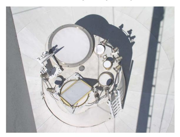
Feed cone needs spot sealed and painted. FE windows are in good condition. Insulation on top of the feed cone has been removed by the site techs. The insulation was retaining water and leaking into the vertex room.
