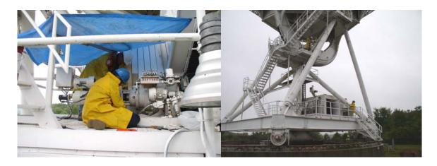
Elevation #1 motor was replaced. Ken and Steve lowering the old motor.
