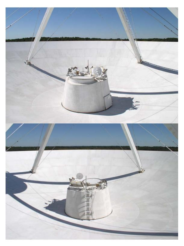
Dish panels are in good condition. Quad legs and guys wire have surface rust. Quad leg bases should be wire brushed and painted with chem-prime. Page 5
