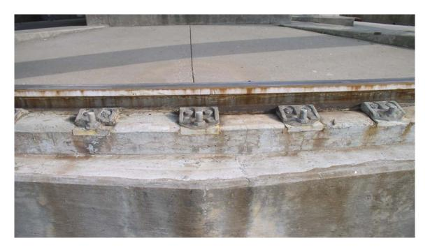
Rail is in good condition. Vulchem is deteriorating off all of the rail clips.
