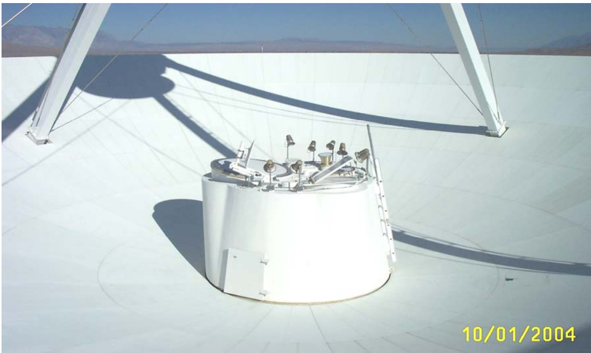
Dish panels, and the panels paint is in good condition. Quad leg paint is excellent. Guy wires are in good condition.
