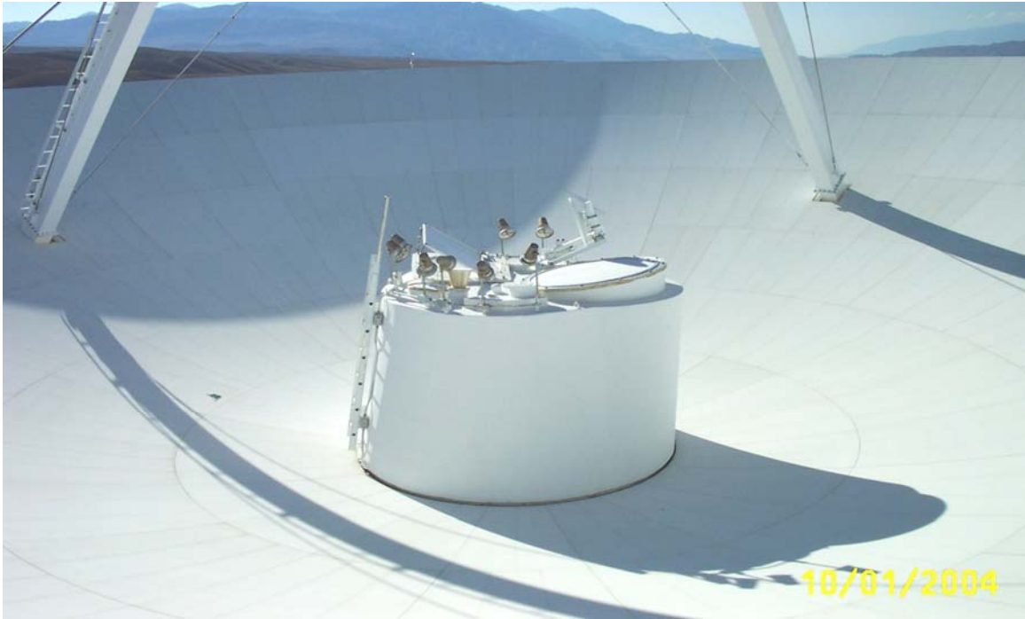
Feed cone was spot sealed and painted with elastomeric.
