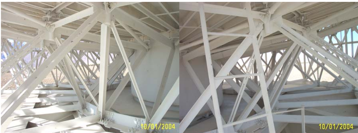
Backup structure paint is in excellent condition.
