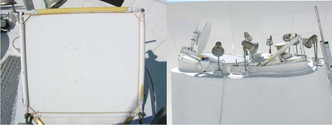
Dichroic reflector is good condition. Elipsoid reflector is in good condition.
