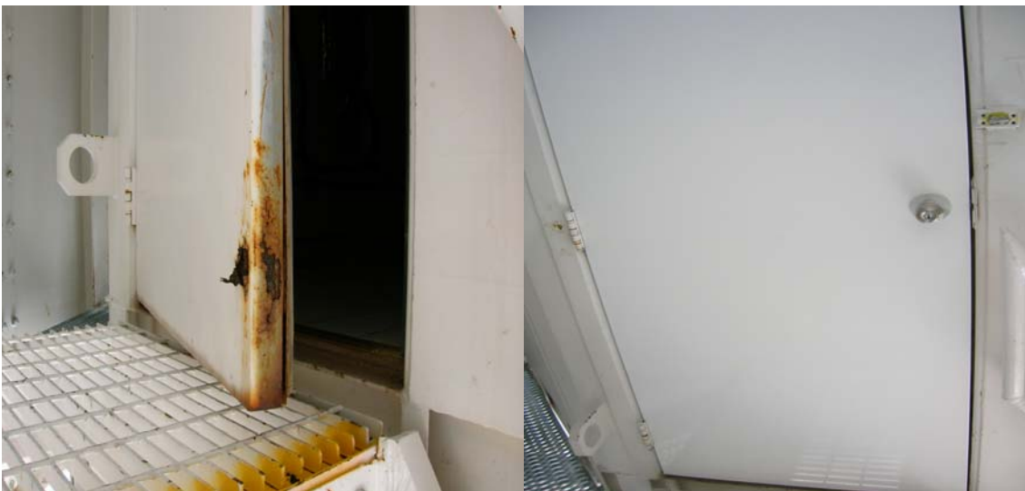
The vertex room door was replaced.
