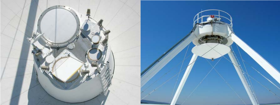
Feed windows & heaters are in good condition. Apex paint is in good shape.
