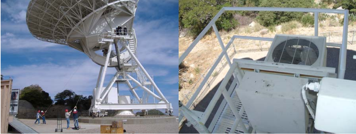
A new HVAC platform extension was installed.
