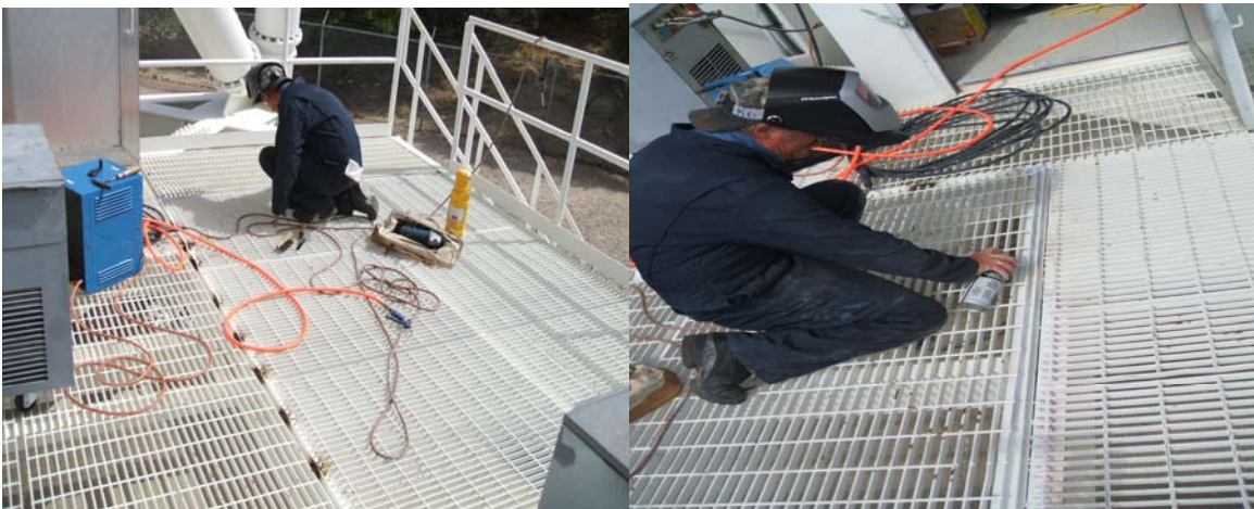
A two inch gap in the pedestal platform grating was repaired.
