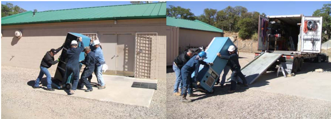
MKIII recorders were replaced by the new MKV recording system. Both MKIII recorders were loaded into the Tiger Team container.
