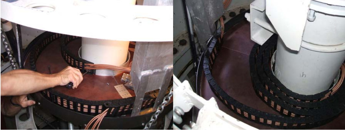
The new Azimuth cable wrap was installed and tested.
