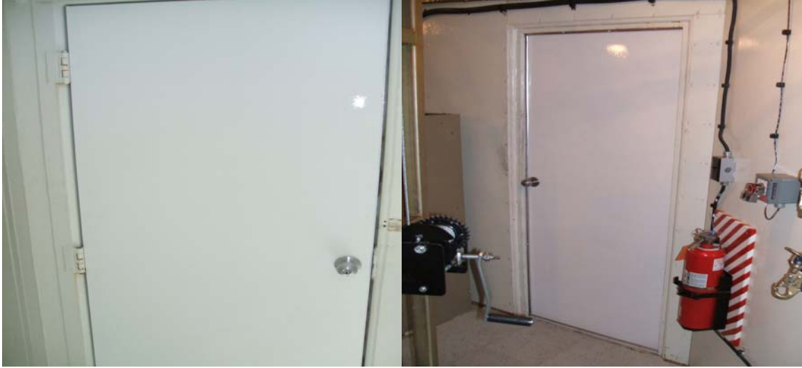
The Vertex room door was replaced.
