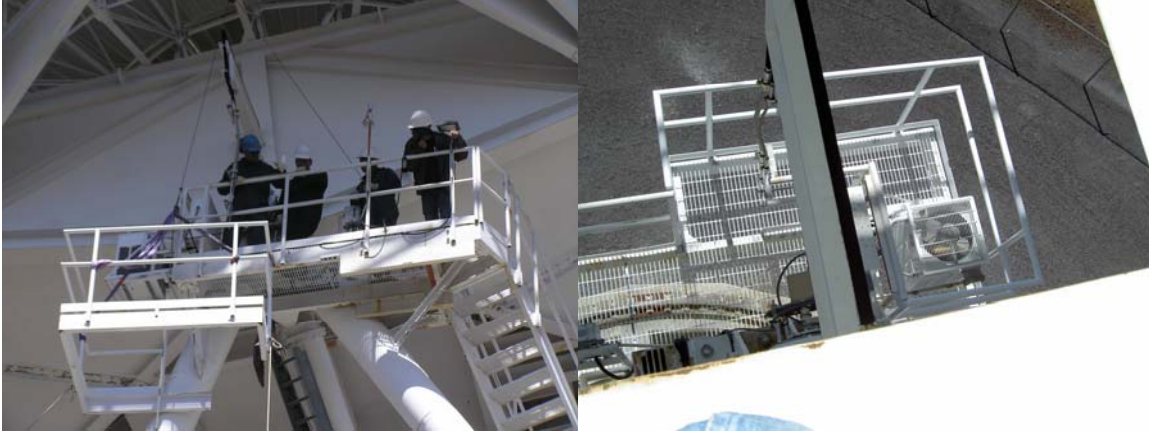
A new Elevation HVAC platform extension was installed.
