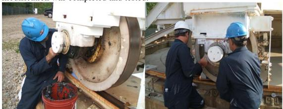
Azimuth wheel bearings were inspected. No AZ bearings were replaced.
