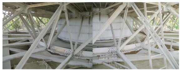
Antenna backup structure is in good condition. Paint is in fair condition.
