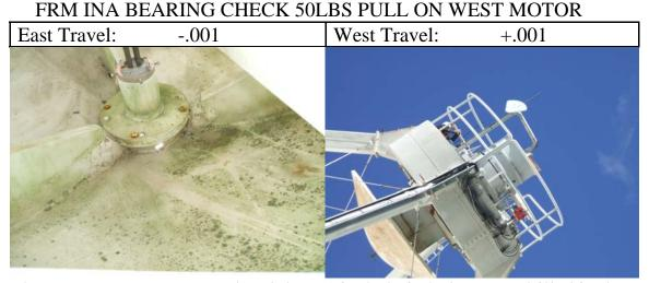
The snow tarp was removed and three 1 inch drain holes were drilled in the center of the sub reflector for drainage. The sub reflector was rebalanced. The rotation single motor modification was also completed.
