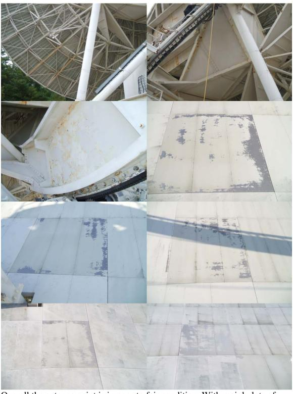
Overall the antenna paint is in poor to fair condition. With mainly lots of surface rust found every where on the structure. The paint on several dish panels is deteriorating.
