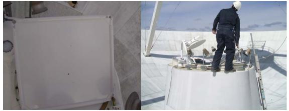
A new dichroic reflector was installed and aligned. The ellipsoid reflector
