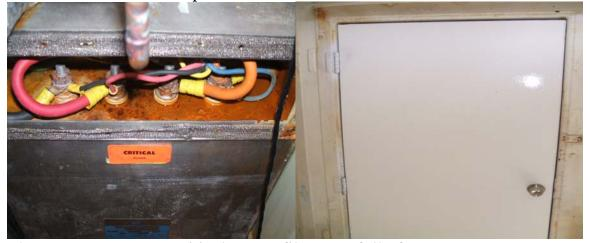
The Vertex room RFI critical power filter was full of water. Vertex room power was shut off. The filter was dried out and connections cleaned. RFI filter leak was located and sealed. The vertex room door was also replaced. Page 8
