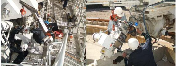
Elevation motors #1 and #2 were replaced. AZ #1 motor needed a new brake assembly. A new blower motor and air box was installed on AZ #2. AZ#2
