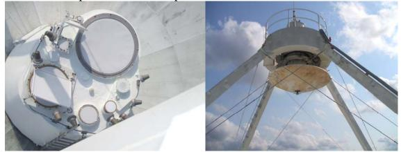
Feed heaters and FE windows are in good condition. Feed heaters operated correctly, 1 feed heater needed replaced. Apex paint is in fair/poor condition.
