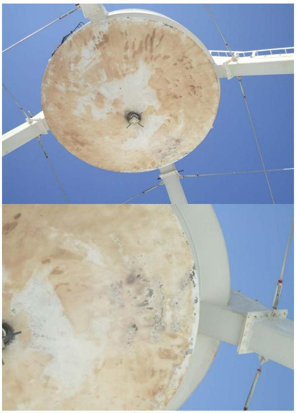
Hancock's sub reflector paint is degrading.
