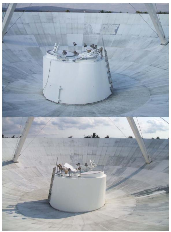
Dish panels are in good condition with no dents. The feed cone was sealed and painted with elastomeric.
