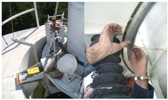
The FRM was given a thorough inspection. The focus flex shaft was replaced along with the INA bearing seal.
