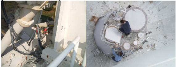
The Elevation synchro side cable wrap was repaired. Vulchem was retaining water on top of the feed cone. The vulchem had to be scrapped off and the feed cone sealed and painted.
