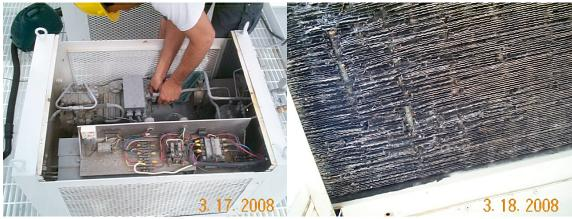
Both CRYO compressors were inspected and are in good condition. Both Contempo condenser coils are deteriorating and will need replaced.
