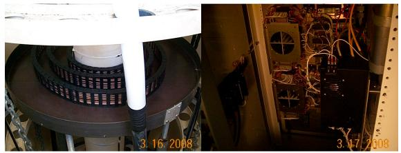
The new IF Cable Wrap was installed and tested. The Site Techs had to install the new drive cabinet power supply shortly before the maintenance team visit due to a failure.
