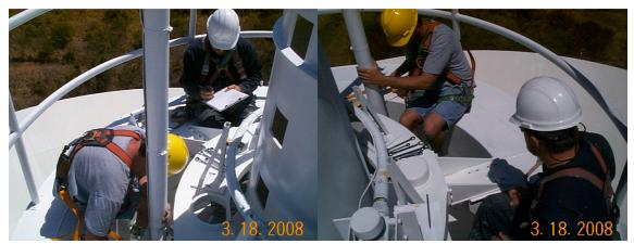
The FRM was given a thorough inspection and the 6 month PM was completed. The focus flex shaft will need replaced in October.
