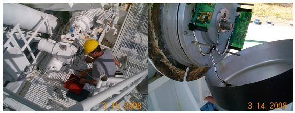
Elevation motor #2 was replaced. Grease was found inside the elevation encoder during the inspection and will have to be replaced.
