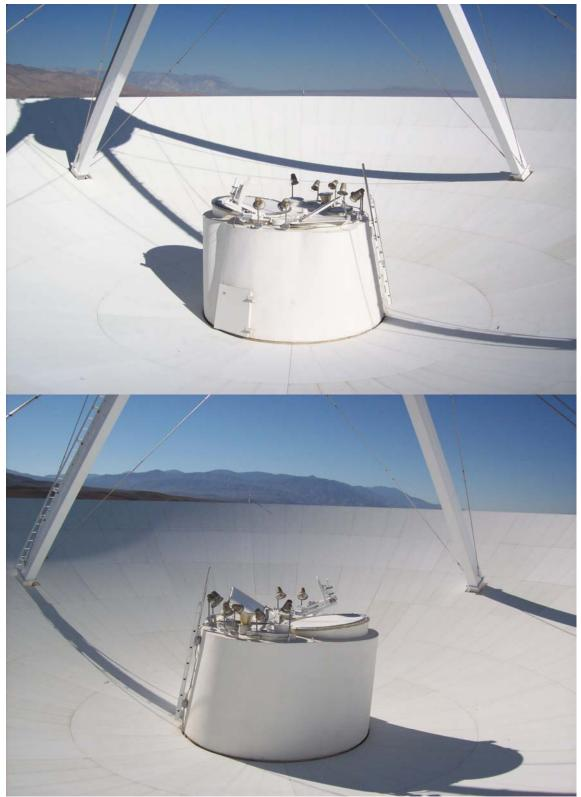
Dish panels are in good condition. The feed cone's elastomeric paint job is holding up well. The feed cone was sealed and painted during the last maintenance trip in 2004. Page 3
