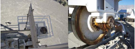
A new Elevation HVAC extension platform was installed. All antenna bearing were inspected.
