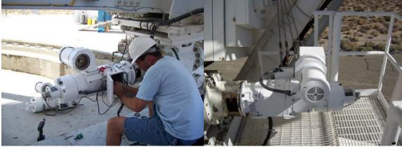
Azimuth #1 and Elevation # 2 motors were both replaced.
