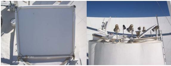
The Dichroic reflector is in excellent condition. The Ellipsoid reflector is in good condition. Ellipsoid actuator operates correctly.
