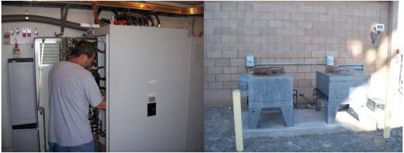
The servo drive cabinet power supply upgrade was completed. The lock out tag out switch tested bad and was replaced. Both Contempo condenser variable speed controllers were replaced after Contempo #2 tested bad.
