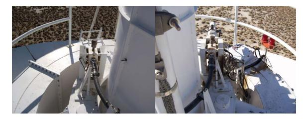
FRM was given a thorough inspection and the focus flex shaft was replaced. Three 1 inch drain holes were drilled in the center of the sub reflector for extra drainage.
