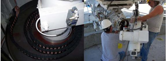
The new IF cable wrap was installed and tested. Azimuth #1 and Azimuth #2 gear box seals were leaking. Both seals were replaced.
