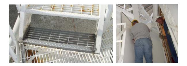
Other badly corroded items such as the step and door shown above were replaced. The new items had paint systems similar to the one on the HVAC platform described above. A finish coat of Acrylic Polysiloxane (Amercoat PSX 1001) was used on the door.
