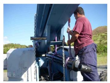
The boom lift cylinder, boom lift cylinder pins and basket cylinder pins were replaced on the Genie S-80 Manlift. These items were supplied by the manufacturer as part of a safety recall. This task was contracted to EM Solutions and was accomplished during the maintenance visit because the task required both a crane and a forklift. A crane and forklift were rented for this maintenance visit as they were needed to facilitate several of the tasks.
