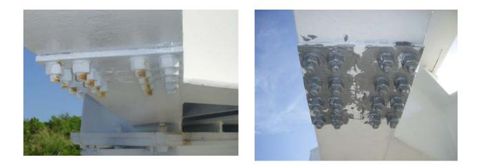
Some of the rust stained bolt heads and nuts were also painted by brush to inhibit further corrosion. Additional stripe painting of bolt heads and nuts should be performed in the near future to deter further corrosion.
