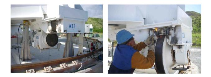
Both azimuth wheel assemblies were replaced during the maintenance period. Azimuth drive # 1 was an old style wheel/axle assembly that was replaced as a preventative maintenance measure. Azimuth drive #2 was a new style wheel/axle assembly that had metal particles in the grease on the inside bearing. This assembly was installed in 2000. This wheel/axle assembly will be disassembled and inspected to establish the cause of the bearing failure.
