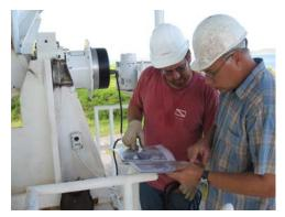
After the new bearing was installed, an improved design encoder mount and a refurbished encoder were mounted and aligned with the elevation axle.
