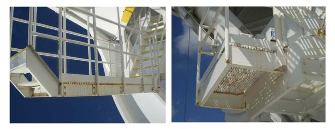
The elevation platform extensions and swinging platform have significant corrosion and will need to be replaced during a future maintenance visit. The hand rails on these parts of the structure are corroding from the inside out. A crane with at least 70 feet of stick will be needed to replace the swinging platform.
