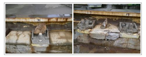
Figure 4: Bolts 31 and 19 before repair
