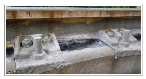
Figure 6: Bolt 91 after grout removal
