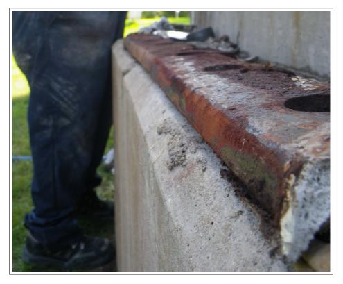
Figure 11: Bent Splice bar from North Liberty antenna
