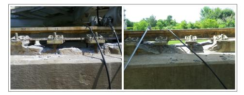
Figure 5: Bolt 72 after grout removal
