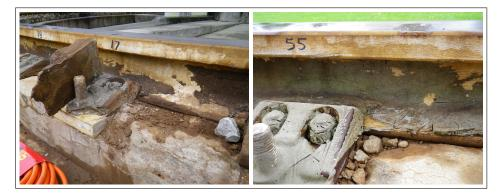
Figure 2: Bolts 17 and 55 before repair
