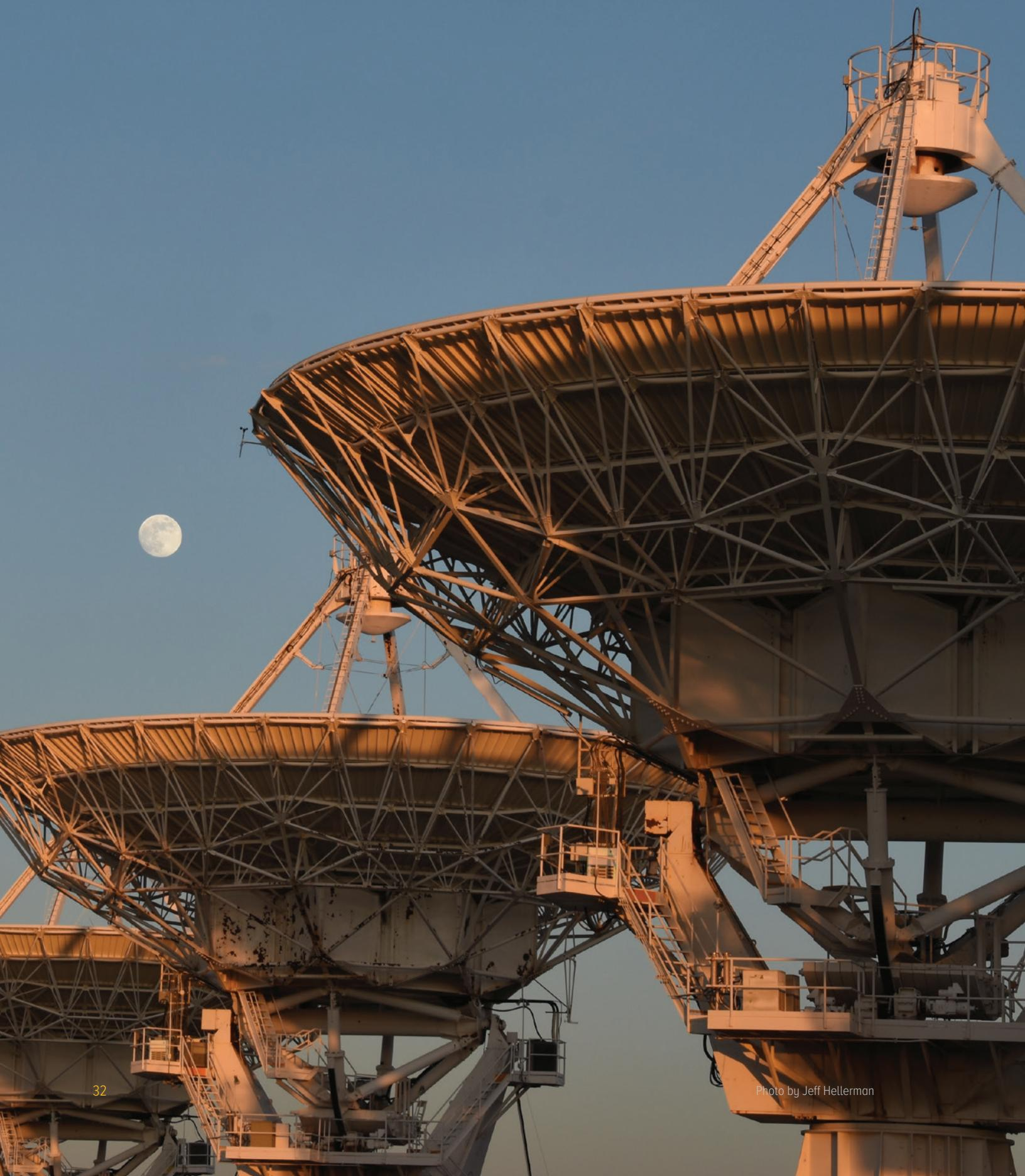
NRAO – New Mexico Operations is responsible for the operation, maintenance, and further development of the Karl G. Jansky Very Large Array (VLA). The Jansky VLA consists of twenty-seven 25-meter diameter antennas laid out in a Y-shaped configuration on the Plains of San Agustin in west-central New Mexico. The original VLA was dedicated in 1980 and has been one of the most scientifically productive telescopes in the world throughout its existence.
