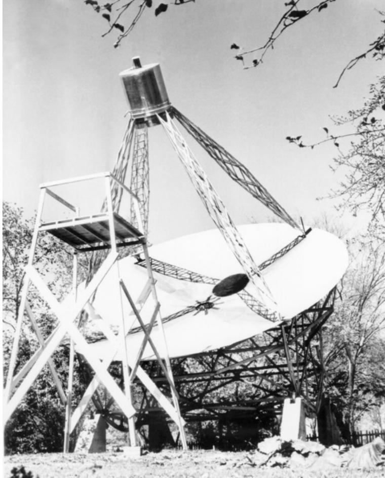
Fig. 4.— Grote Reber's backyard radio telescope in Wheaton, IL. The parabolic reflector is about 10 m in diameter.
