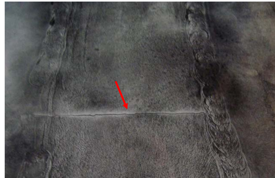
second welding joint
