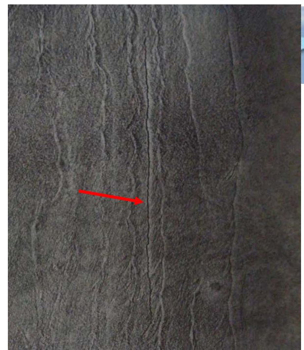
first welding joint
