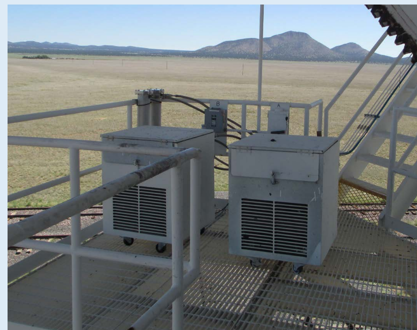
Figure 5: Helium compressors Mounted on VLA antenna
